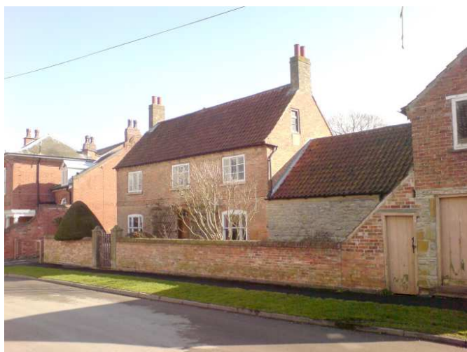
Granby Farmhouse, Church Street (grade II)
